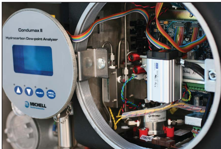
Figure 6 Removal of Interface/Display
